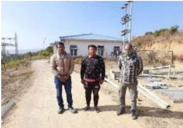
132/33 kV Ukhrul Sub-station
