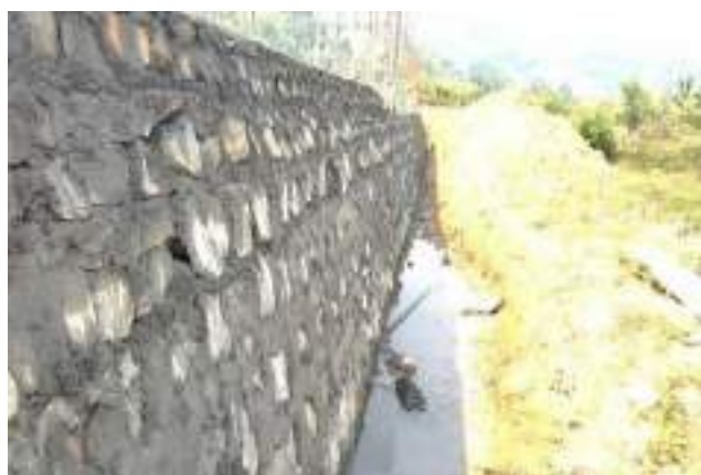
RRM Wall at 33/11 kV Andro S/S
