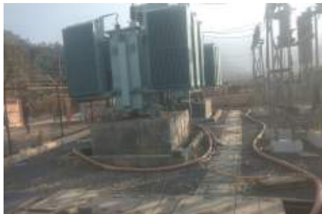
Stone Pitching at 33/11 kV Sanjenbam S/S
