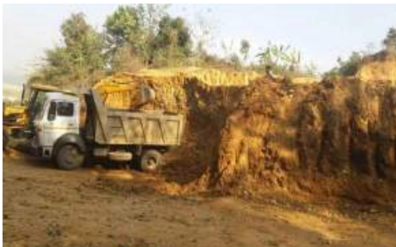
Borrow Site for Andro Substation
