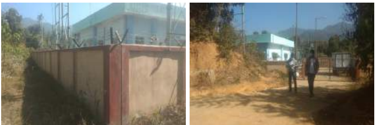
Boundary Wall and Gate at 33/11 kV Tuilaphai Substation
