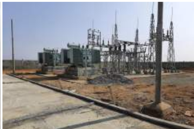
Stone Pitching at 33/11 kV Andro S/S
