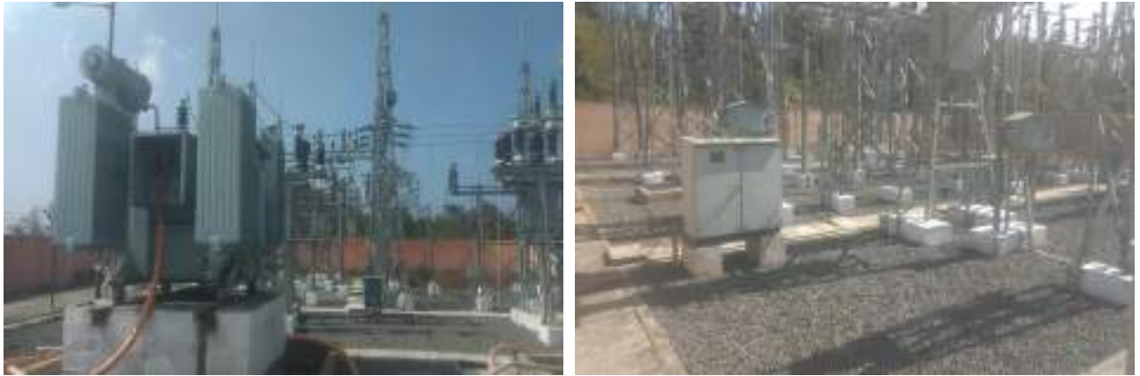
Levelled surface at 33/11 kV Thangal and Tuilaphai Substations
