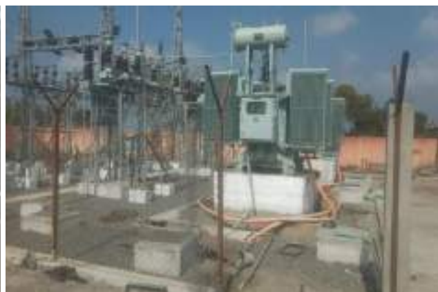
Stone Pitching at 33/11 kV Thangal S/S
