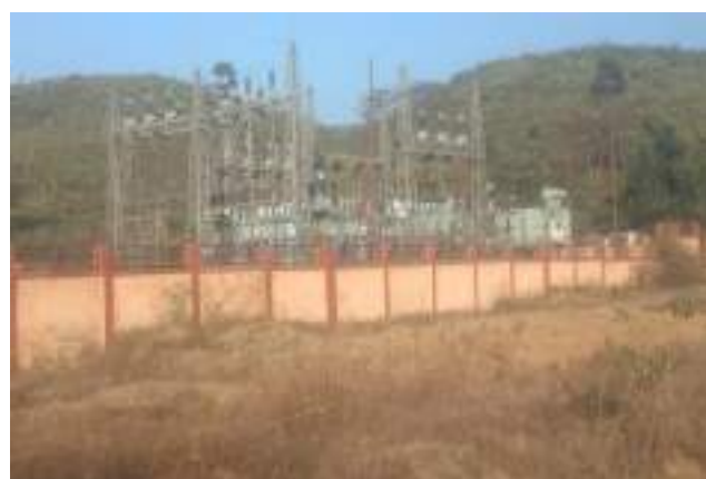
Retaining Wall at 33/11 kV Sanjenbam S/S
