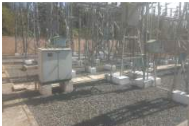
Stone Pitching at 33/11 kV Tuilaphai S/S
